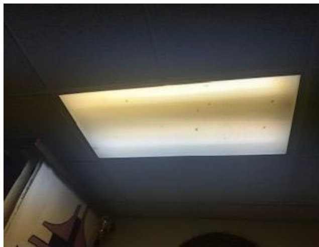
Classroom lighting before changes.
