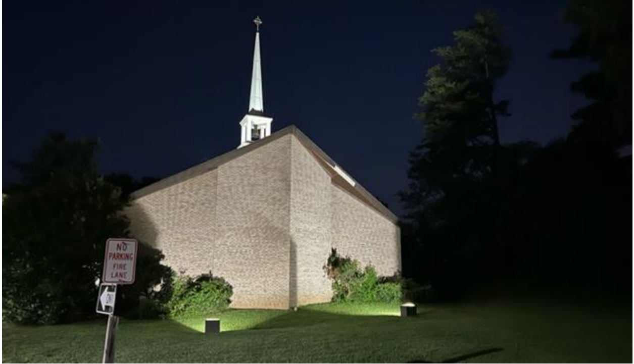
Improved lighting added to the front of the church.
